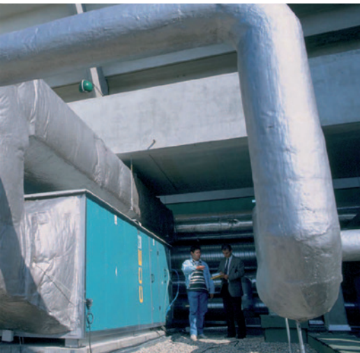
Circulating pumps for building management
